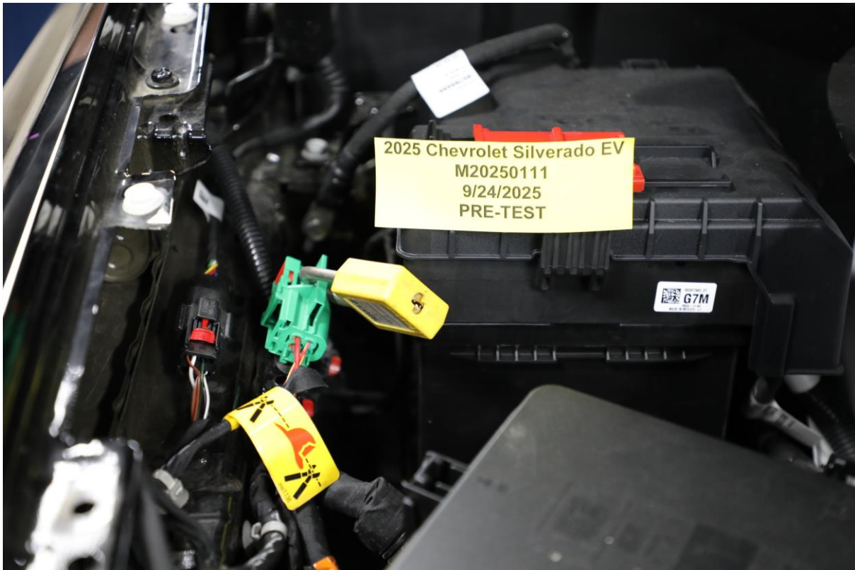
305-08 Manual High Voltage Service Disconnect Removed
